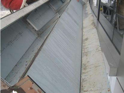
Condensation Observed at Inboard Face of Metal Panel Cladding Elements
