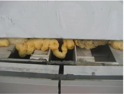
Air/Moisture Barrier Tie-in Found to be Discontinuous at Opaque Wall-to-Glazing System Interface
