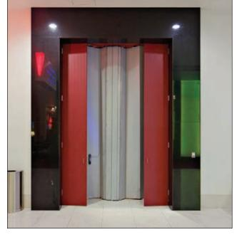
CASE 2: Side Acting Accordion with Complying Swing Egress Door & Vertical Acting with Complying Swing Egress Door(s)
