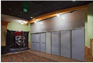
CASE 2: Vertical Coiling without Egress, Vertical Acting with Complying Swing Egress Door(s) & Side Acting without Egress
