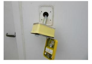
Construction Issue: Discontinuous Air Barrier
