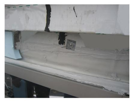
Air/Moisture Barrier Tie-in Made Continuous at Opaque Wall-to-Glazing System Interface
