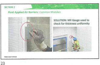
SECTION 2 Fluid Applied Air Barriers: Common Mistakes Shrinkage-Cracking Sealing of Penetrations CONTINUITY IS COMPROMISED
